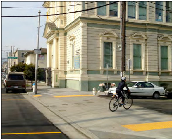
RAISED CROSSWALK WITH FEATURE PAVING
