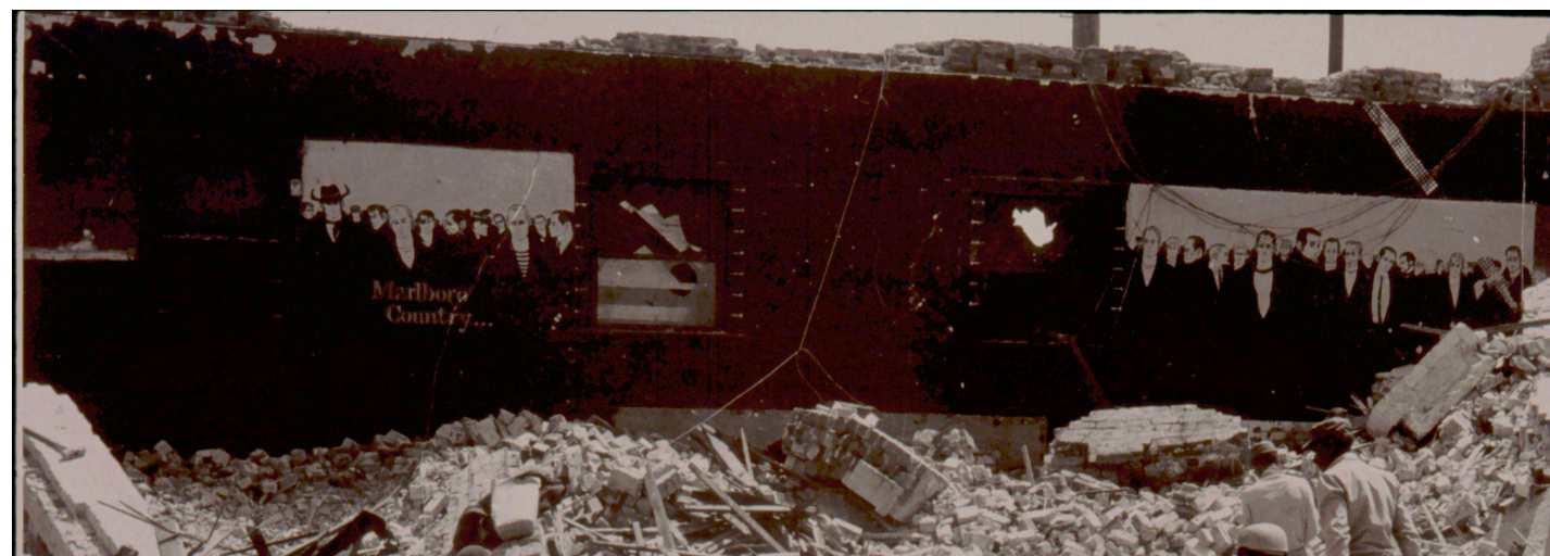
THE TOOL BOX: MID DEMOLITION
